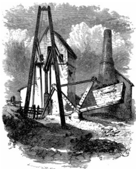
CARDOZOS PUMPING-ENGINE, UNITED MINES.
