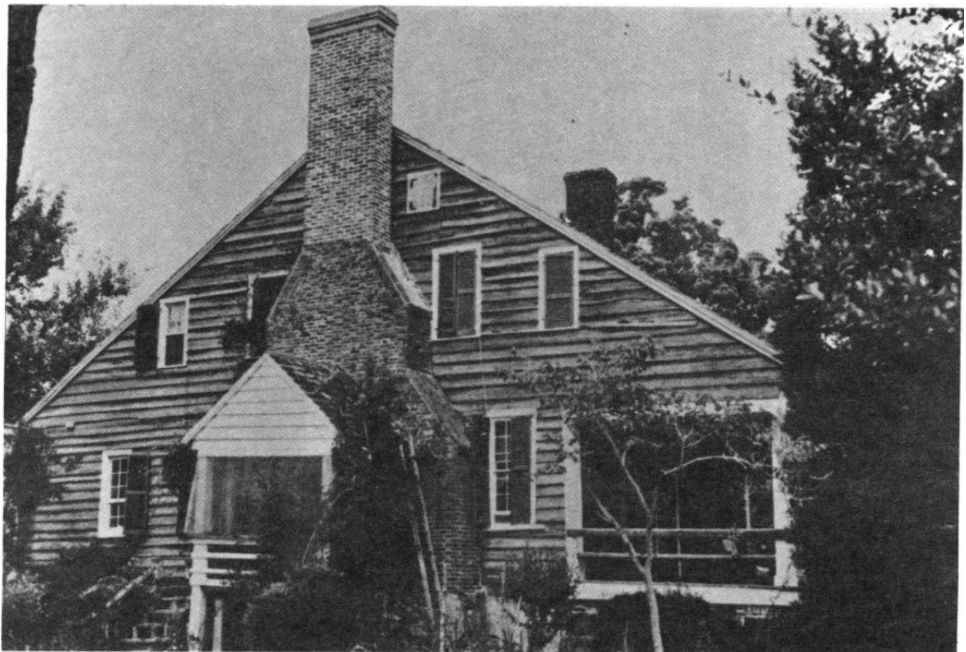
FIGURE 52. THE SLOOP POINT HOUSE.
