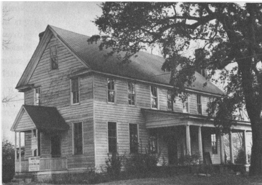
FIGURE 11. THE PALMER HOUSE BEFORE RESTORATION.
