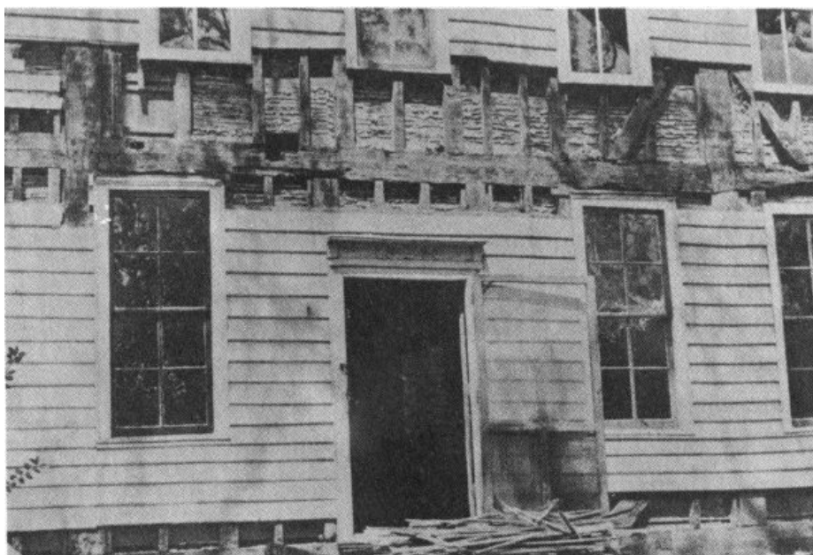
FIGURE 28. THE PALMER HOUSE, BATH, DURING RESTORATION.
