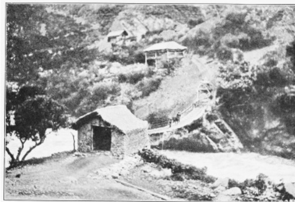
THE TOLL BRIDGE OF TABLACHACA
