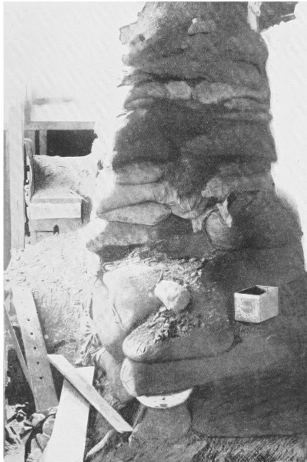
At the tunnel mouth.
