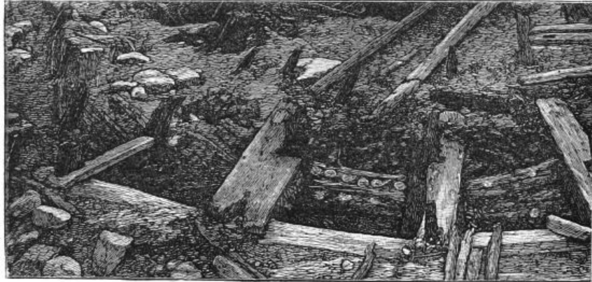
Fig. 190.—Portion of north side of Crannog, with the space between inner and second circle of piles dug out, showing arrangement of Transverse Beams and structure of the Log Pavement. (From Photograph by Mr. Lawrie.)
