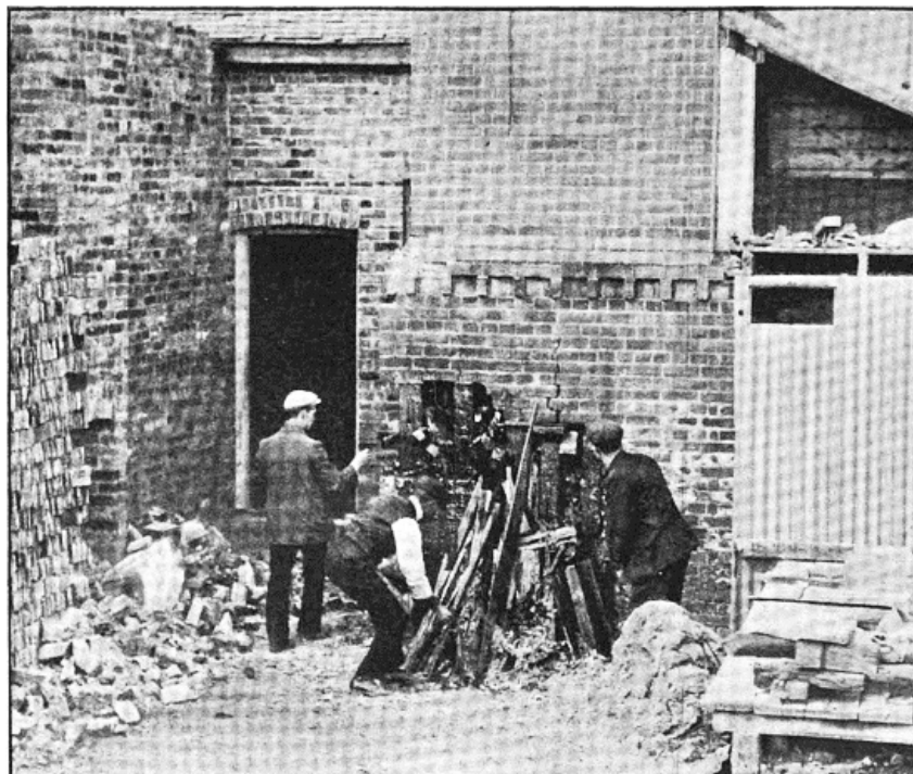
THE OLD-FASHIONED METHOD OF BURNING PROPS—APPLYING THE MATCH TO THE MATERIAL. WHEN THE SUPPORTS HAVE BURNT THROUGH
