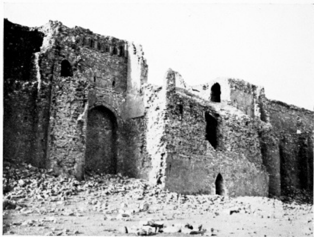
Fig. 87.—UKHEIDIR, NORTH GATE, FROM OUTSIDE.
