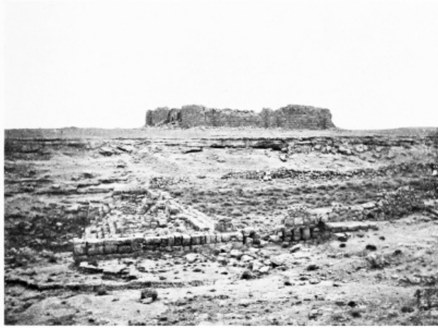
Fig. 64.—KAŞR KHUBBÂZ AND RUINS OF THE TANK.
