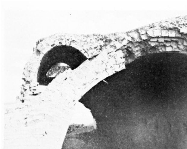
Fig. 133.—KHÂN KHERNÎNA, VAULT, SHOWING TUBE.
