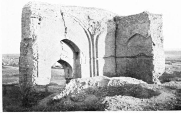
Fig. 44.—RAQQAḤ, INTERIOR OF BAGHDĀD GATE.
