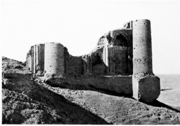
Fig. 144.—SÂMARRĀ, EL 'ASHIḲ, WEST END OF NORTH FAÇADE.
