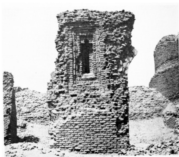
Fig. 166.—ABU DULÂF, NICHED PIER OF NORTHERN ARCADE.
