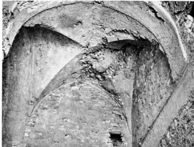
Fig. 98.—UKHEIDIR, GROIN IN CORRIDOR C.
