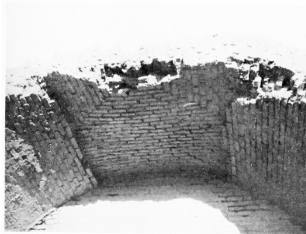
Fig. 132.—KHÂN KHERNÎNA, DETAIL OF FLAT VAULT.
