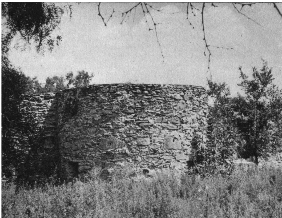
A fortified tower has thirty-six-inch walls. Holes for cannon muzzles were created near the base. Musket loopholes can be seen higher.
