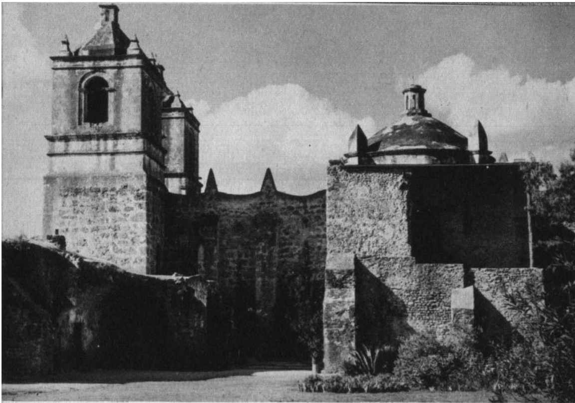
Conception from the south side presents the Moorish dome with its wide stone serrations. The walls at the right are all that remain of the mission kitchen, destroyed during the battle of Conception in 1835.
