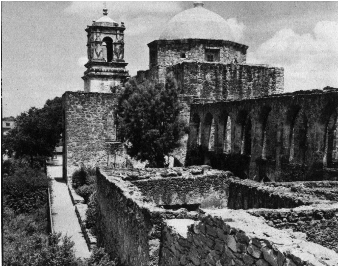
Two-story cloisters connect with the main building.
