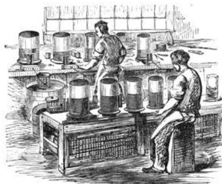
Fig. 409.—Fine wire-drawing.
