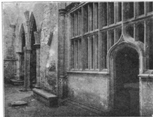
THE NORTH CHAPEL AISLE.
