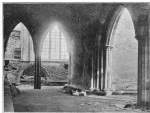
VIEW LOOKING N. IN ANTE-CHAPEL TO LADY CHAPEL.
