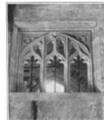
RECENTLY DISCOVERED WINDOW IN BISHOP VAUGHAN'S CHAPEL.
