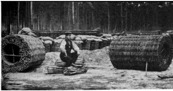
Constructing gabions for the attack on Petersburg. When filled with earth, these cylindrical, basket-like objects offered strong protection against enemy fire.
