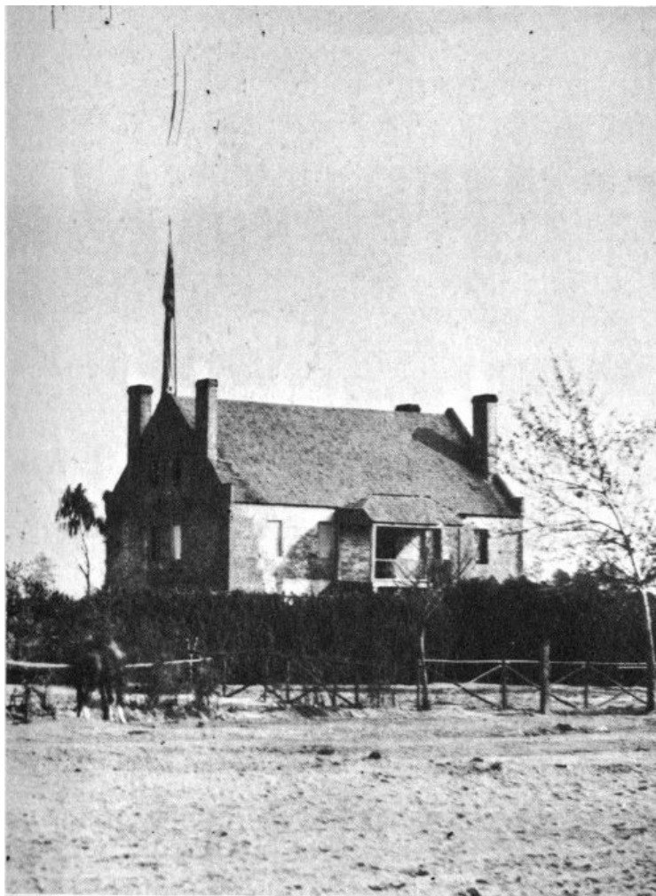
Globe Tavern, near the Weldon Railroad. During the Battle for the Weldon Railroad, August 18-21, 1864, this building was headquarters for Maj. Gen. Gouverneur K. Warren's V Corps.
