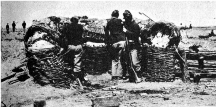
Federal pickets in front of Union Fort Sedgwick, opposite Confederate Fort Mahone. Note how the gabions are being used.
