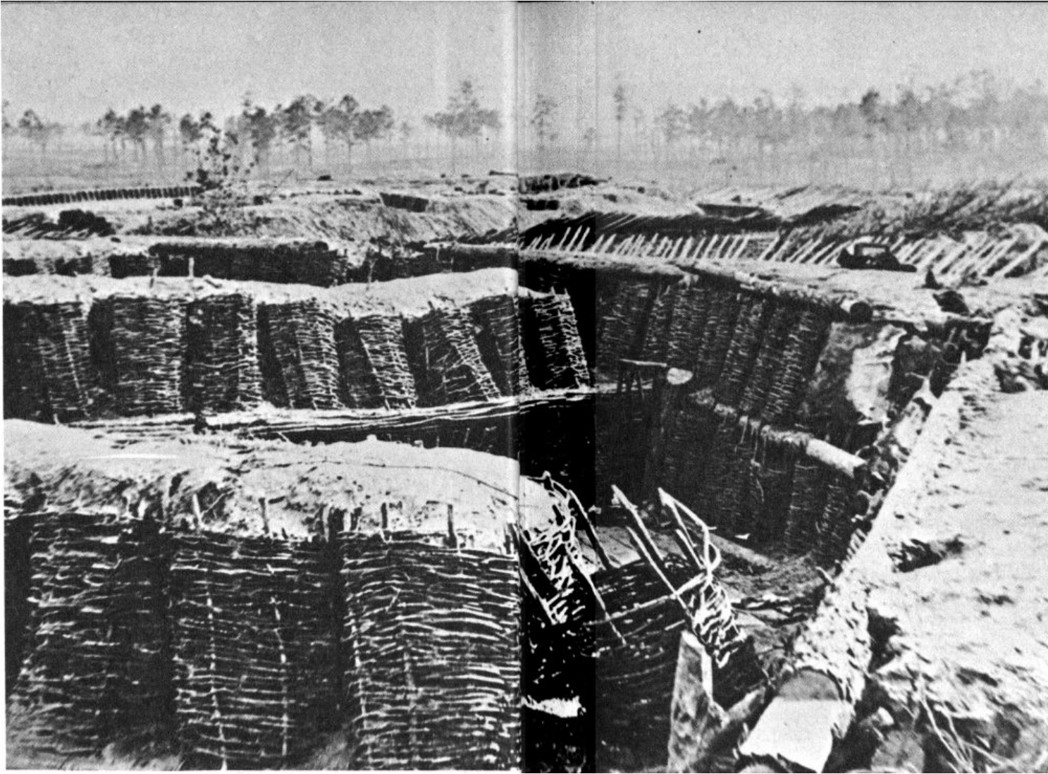
A section of the Confederate defense lines around Petersburg. Note the use of wickerware (gabions), sharpened stakes (fraises), and branches (abatis) to protect the position.
