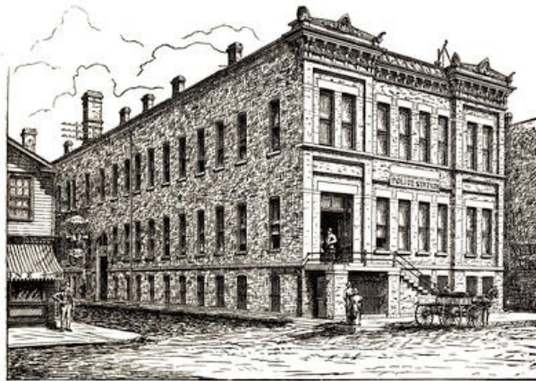
THE DESPLAINES STREET STATION.
