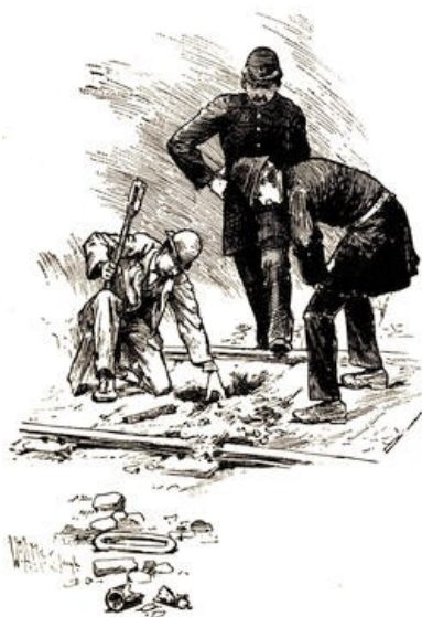
A DANGEROUS STORING-PLACE.
