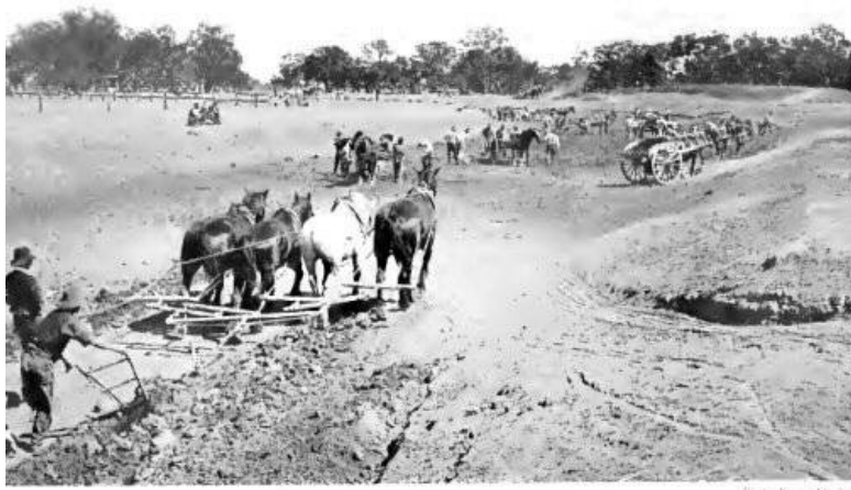
EXCAVATING AN IRRIGATION CHANNEL.
