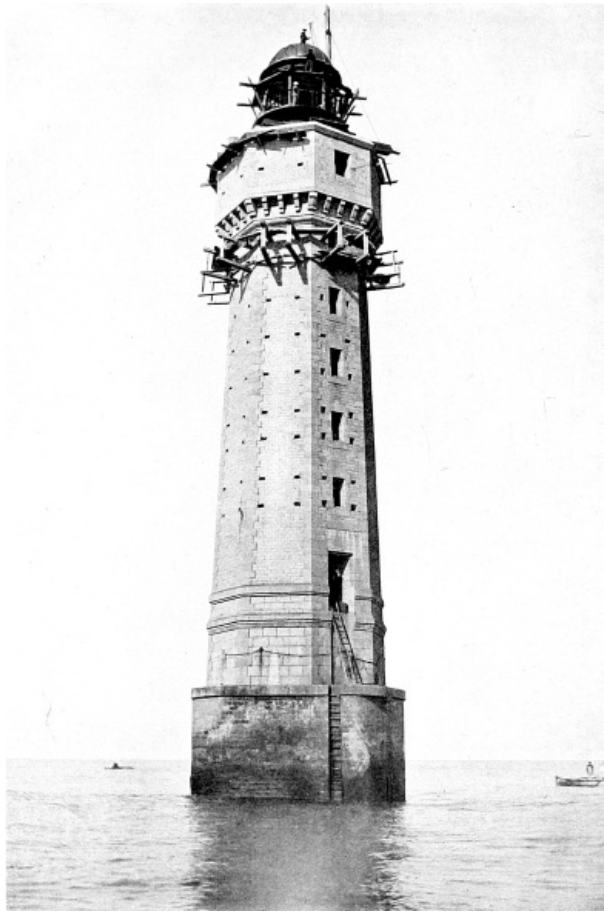
FITTING THE LANTERN OF LA JUMENT LIGHT.
