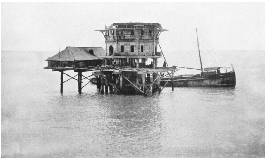
THE ONE FATHOM BANK LIGHTHOUSE, MALACCA STRAITS, IN COURSE OF ERECTION.
