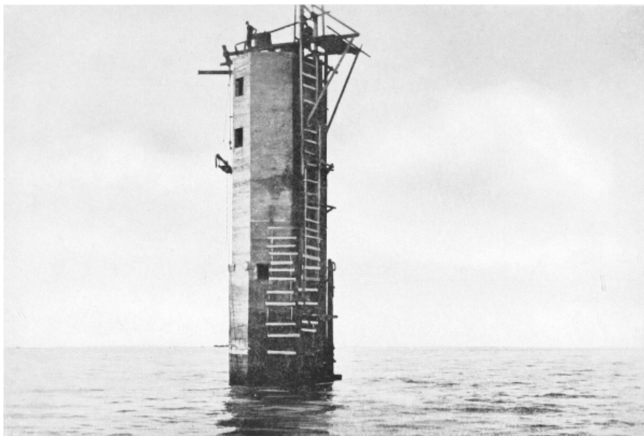
THE PLATTE FOUGÈRE LIGHTHOUSE UNDER CONSTRUCTION.
