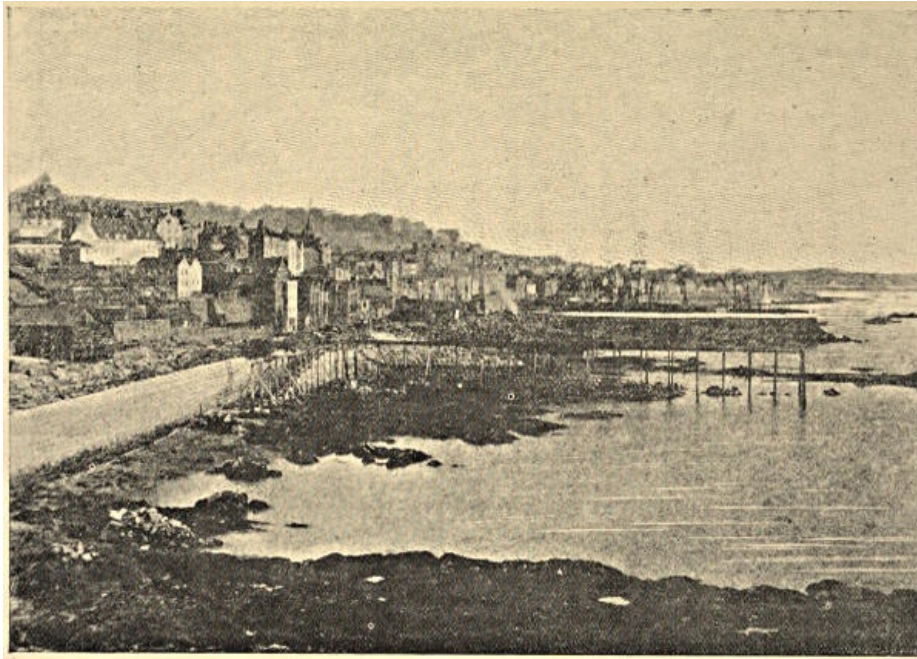
Building the south arm of the Town Harbour, connecting Castle Cornet with the Island.
