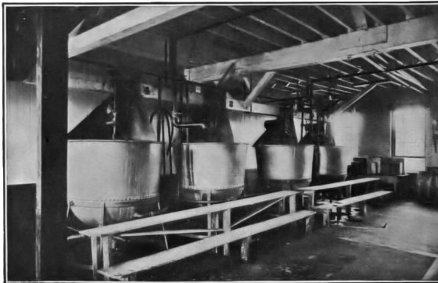
FIG. 3.—A section of a kitchen showing the copper cookers.
