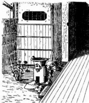
Fig. 237.—Verandah showing swinging closet for rain-doors, and also Chōdzu-bachi.
