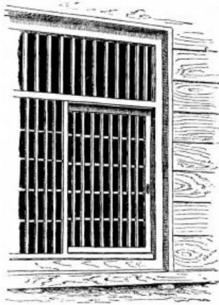
Fig. 225.—Grated entrance, with sliding door.
