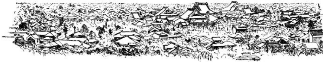
Fig. 2.—View in Tokio, showing temples and gardens. (Copied from a Photograph).
