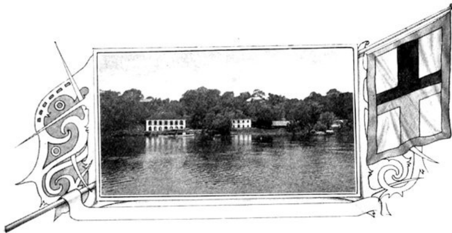
THE BORNEO COMPANY'S OFFICES, KUCHING.
