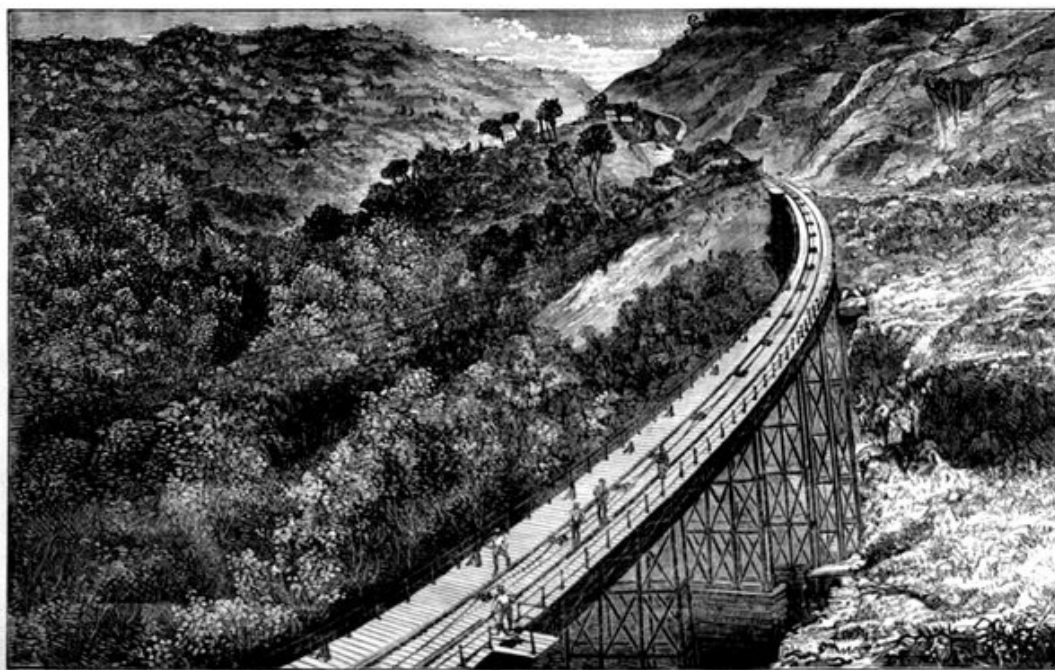
Bridge Viaduct on the San Paulo Railway.
