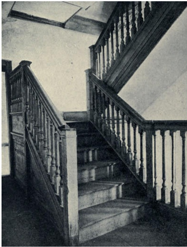
Illus. 421.—Stairs at “Graeme Park,” Horsham.
