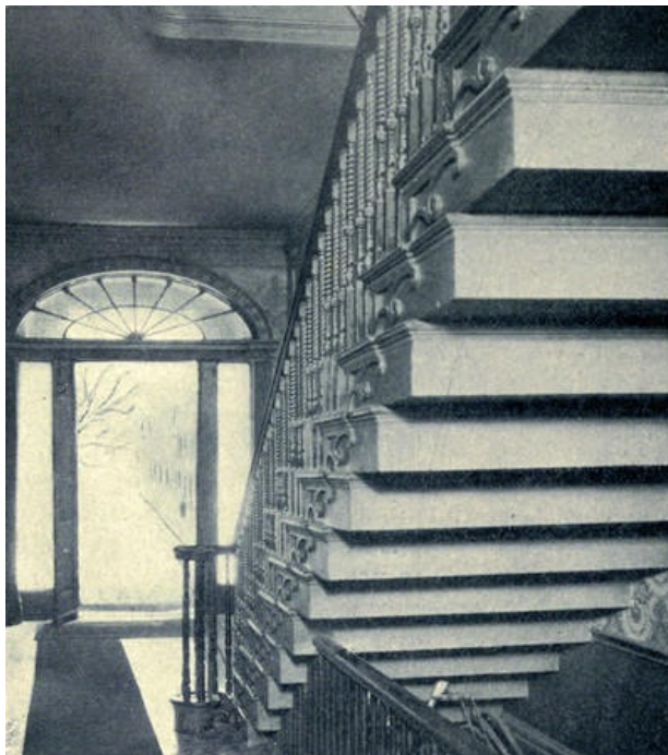
Illus. 404.—Stairs in Harrison Gray Otis House, Boston, 1795.
