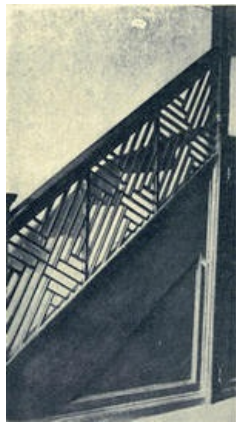
Illus. 426.—Fretwork Balustrade, Garrett House, Williamsburg.
