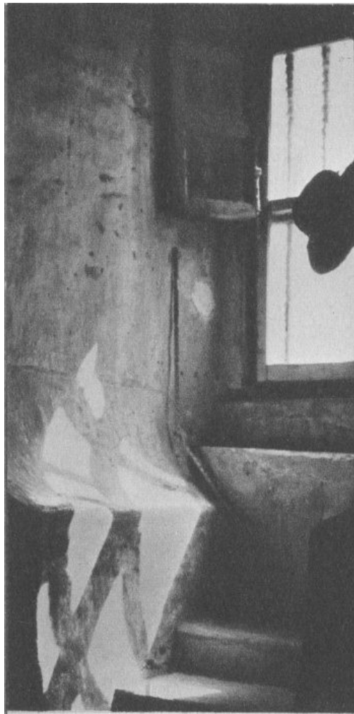
DETAIL OF BAPTISTRY WINDOW.
