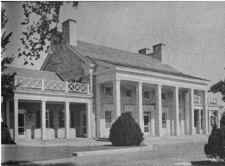
Park Administration and Museum Building.
