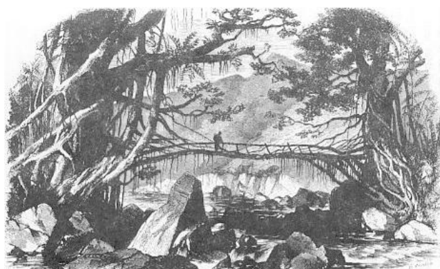
"Living bridge" formed of the aerial roots of the India-rubber and other kinds of figs
