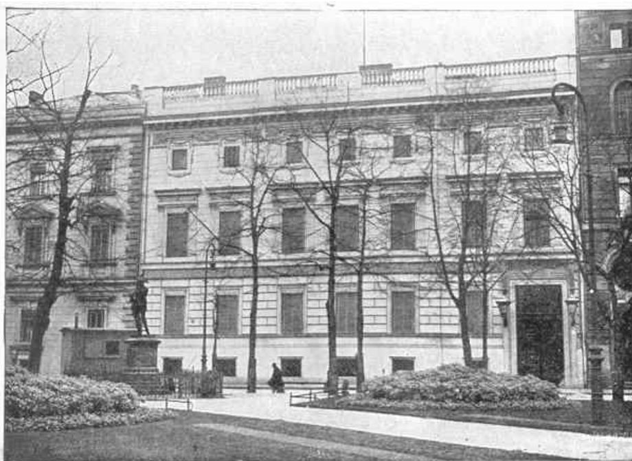
THE HOUSE ON THE WILHELM PLATZ, RENTED FOR USE AS THE EMBASSY.
