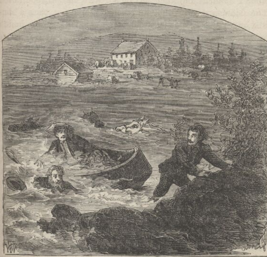
CROSSING THE FLOOD.
