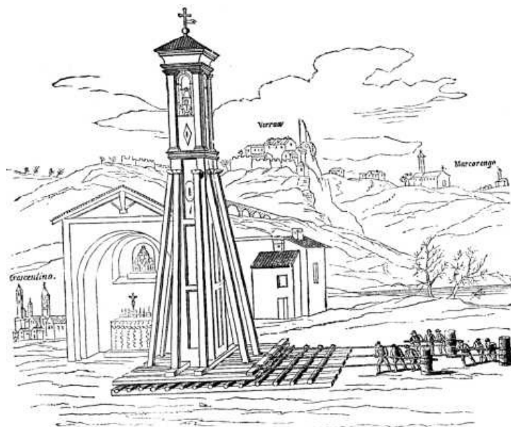
FIG. 1.--REMOVAL OF A BELFRY AT CRESCENTINO IN 1776
