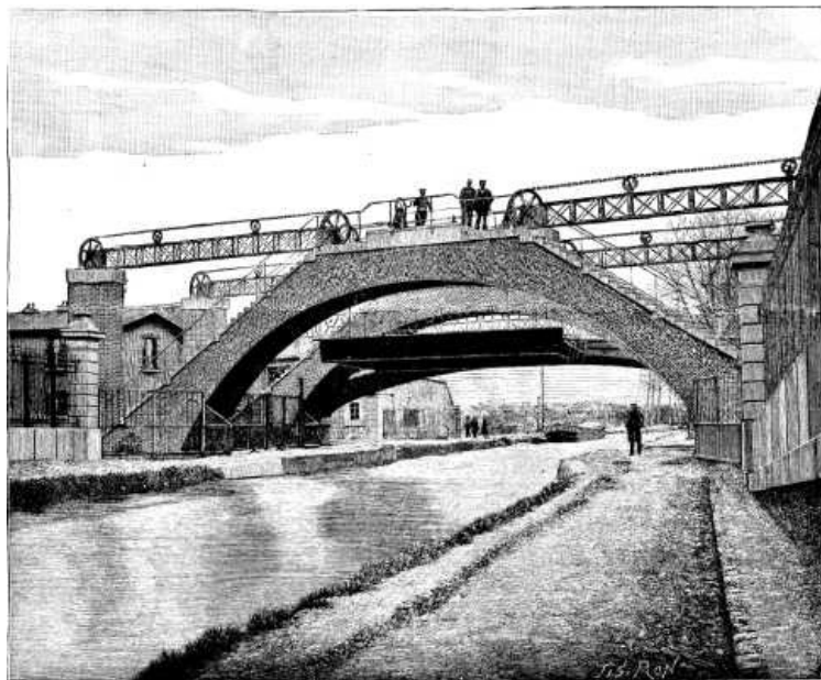
FIG. 1.--LIFT BRIDGE OVER THE OURCQ CANAL.
