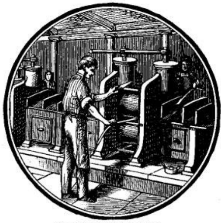
ROLLING THE STEEL.
