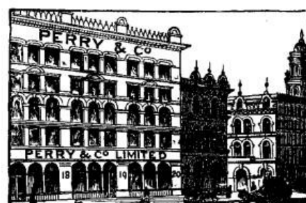
LONDON HOUSE, HOLBORN VIADUCT.
